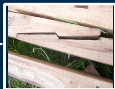
Use proper splice joinery
