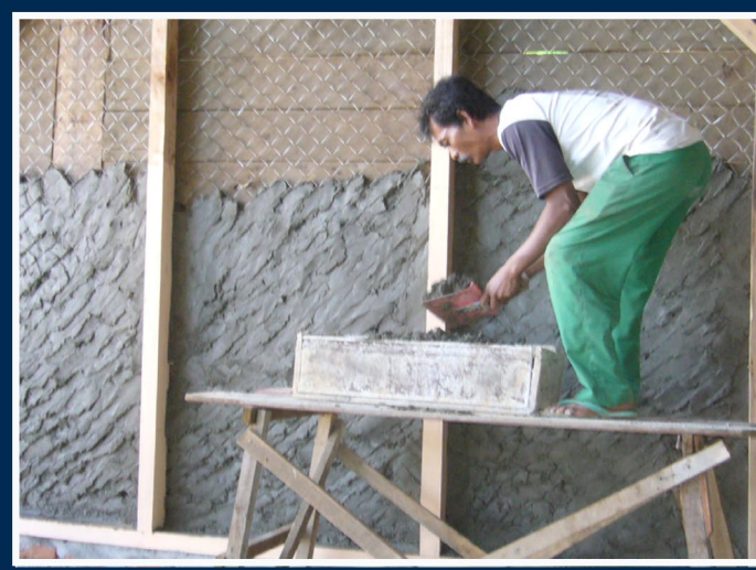
Install backing boards and plaster
